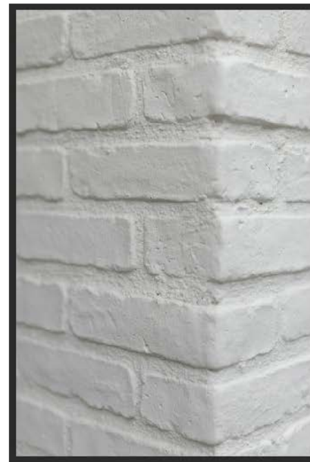
PAINTED BRICK TO MATCH SW7077
